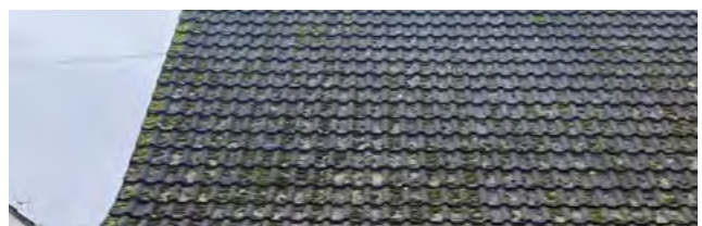
Concrete interlocking tiling
