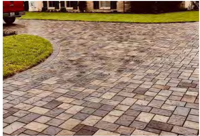
Figure 56: A good example of permeable paver (Source: https://www.paverconnection.com/testimonial/hedwig-village-permeable-driveway-and-patio-upgrade/ )
