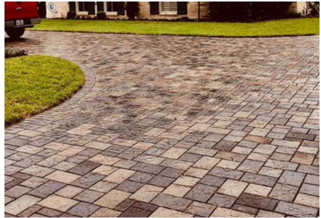
Figure 54: A good example of permeable paver (Source: https://www.paverconnection.com/testimonial/hedwig-village-permeable-driveway-and-patio-upgrade/ )
