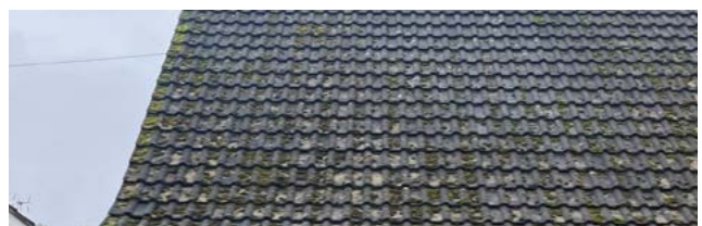
Concrete interlocking tiling
